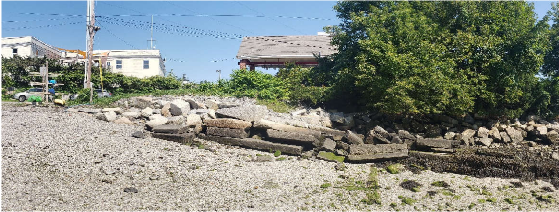
Figure 2: Existing kayak rack and Living Shoreline location
