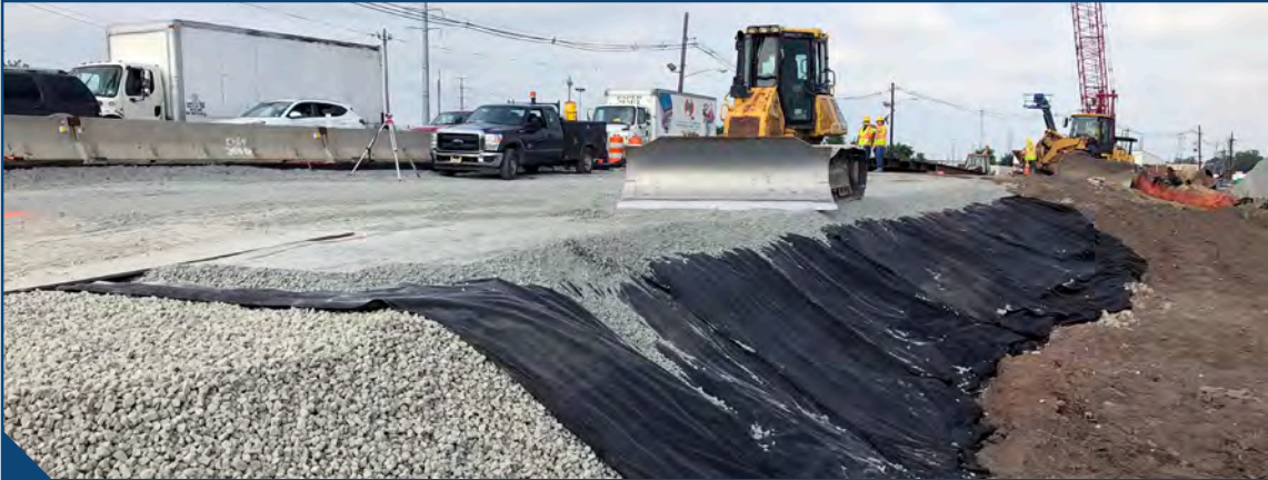
FIG. 4: Placement of capping material on UL-FGA.
