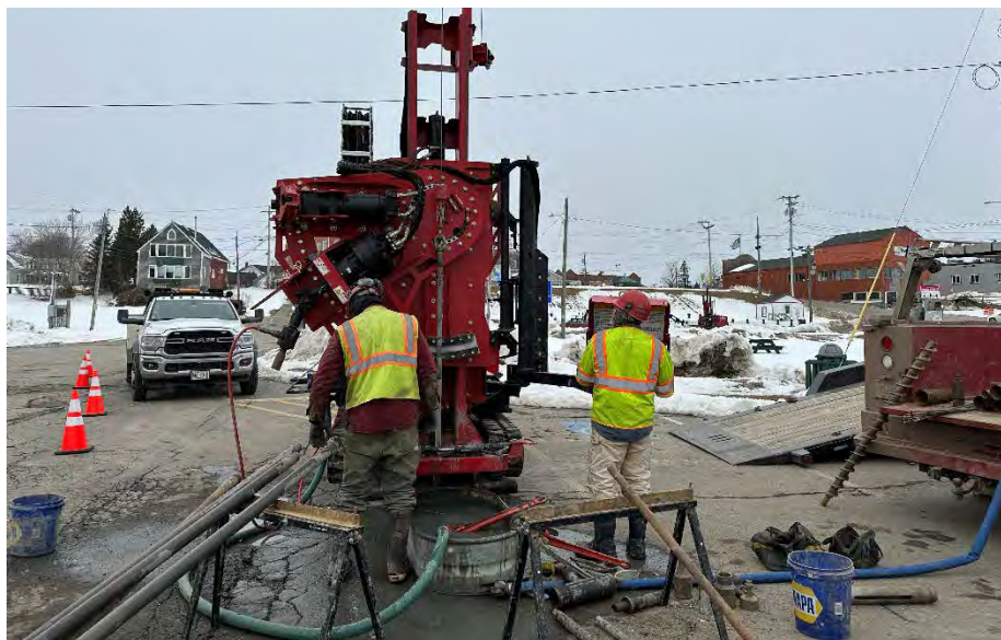
Rotary Wash w/Casing at Test Boring B-4
