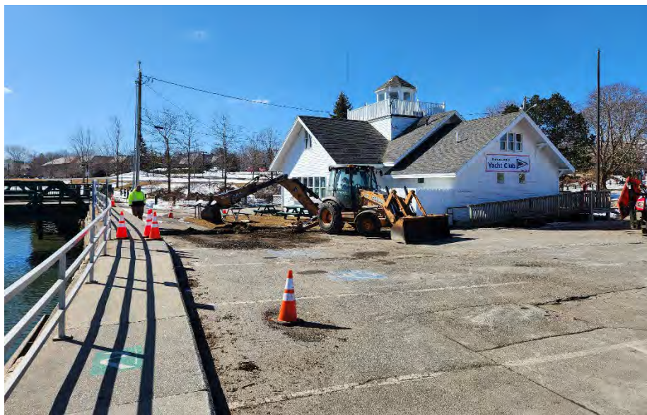
Excavation of Test Pit TP-2
