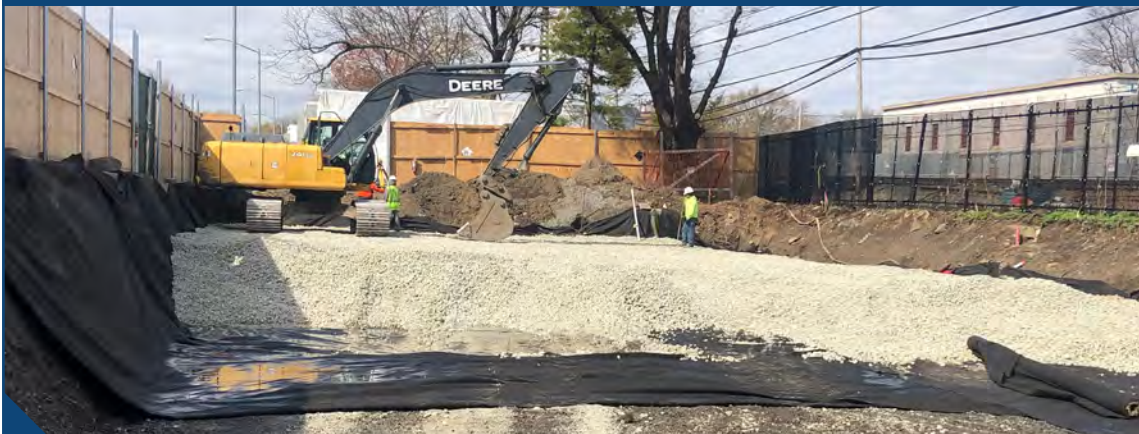
FIG. 3: Compaction of UL-FGA with an excavator.
